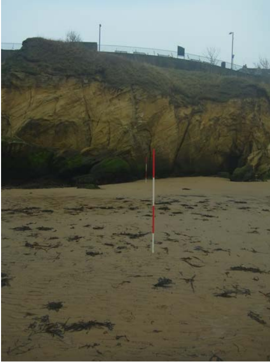
Plate 3 – Survey photograph 1aNTDC05_20140403_Up3.JPG
