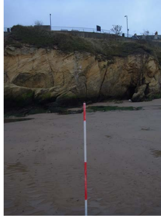
Plate 4 – Survey photograph 1aNTDC05_20131018_Up3.jpg
