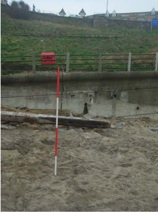
Plate 7 – Survey photograph 1aNTDC08_20140403_Up2.JPG
