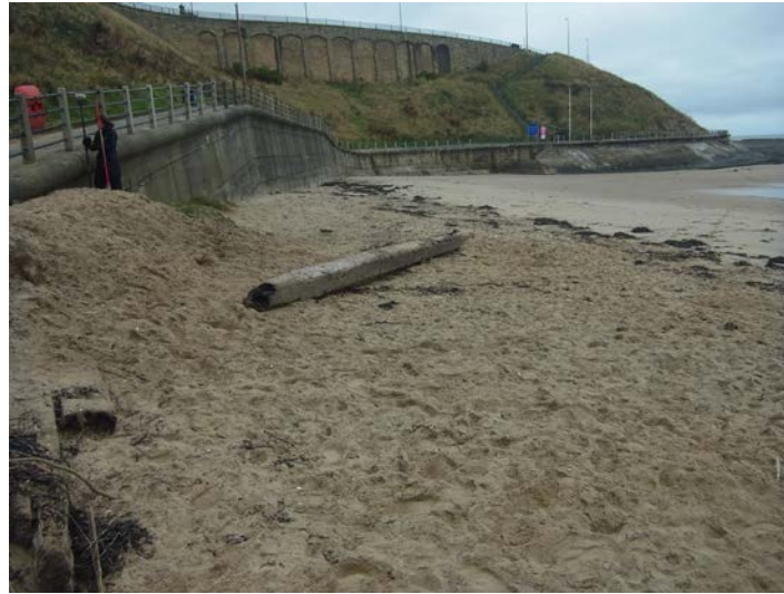
Plate 8 – Survey photograph 1aNTDC08_20131018_N2.JPG.
