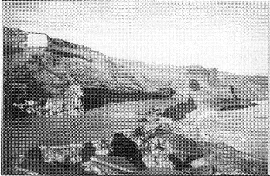
*Figure 6.2 Damaged defences at south end of Tenant's Cliff*
